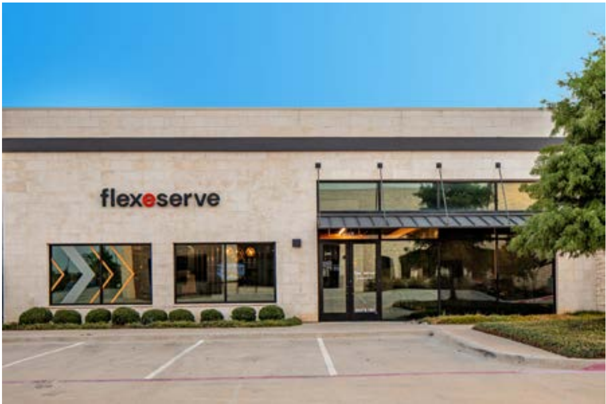
Flexeserve's HQ and Culinary Support Center in Southlake, Dallas, TX
